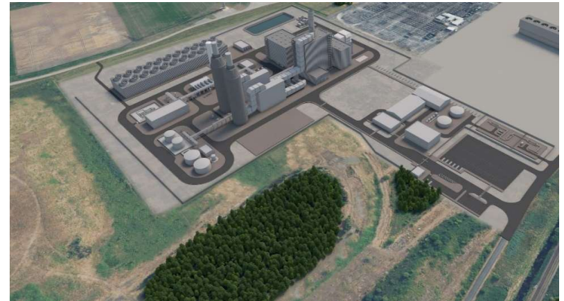
Figure NTS5: Visualisation of the Proposed PCC Site based upon maximum dimensions and twin absorbers
